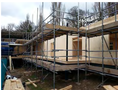
Installation phase two
