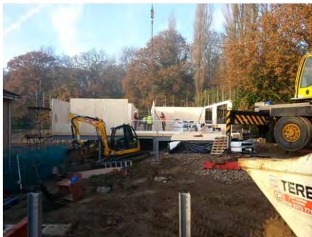
Installation phase one
