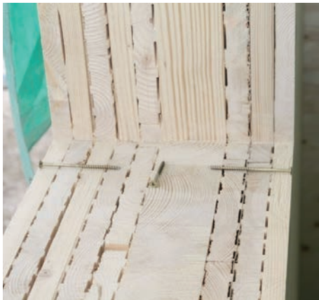
Wood 100 Exterior Wall. Crosswise layered dried lumber planks are connected with beech dowels only. Through the only use of wood the construction reaches health and ecological benefits which outweigh any other building style compared in a long term run.
