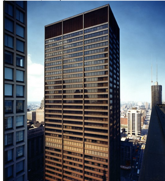
Abb. 118: C.F. Murphy Associates, Richard-Daley-Center, Chicago, 1963-65 ( https://www.som.com , Stand: Februar 2019)
