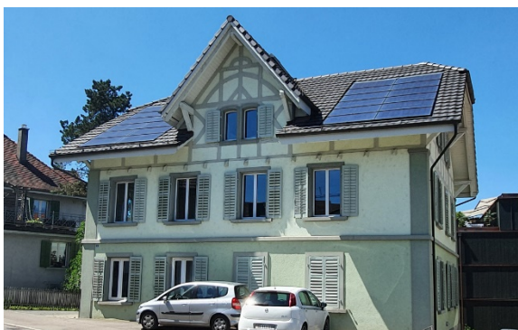
Abb. 48, Indachanlage in Muri
